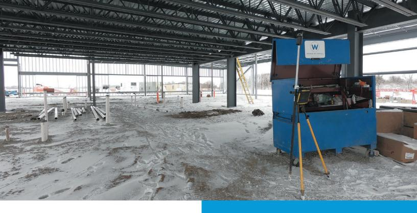
One of Riddell's favorite features of the X7 scanner is the Trimble Registration Assist for in-field registration that allows for automatic scan orientation and alignment with the last pre-selected scan. He also likes the ability to customize the scanner to allow for faster scans and the ability to view both scans and 3D models on the tablet controller for onsite viewing.
