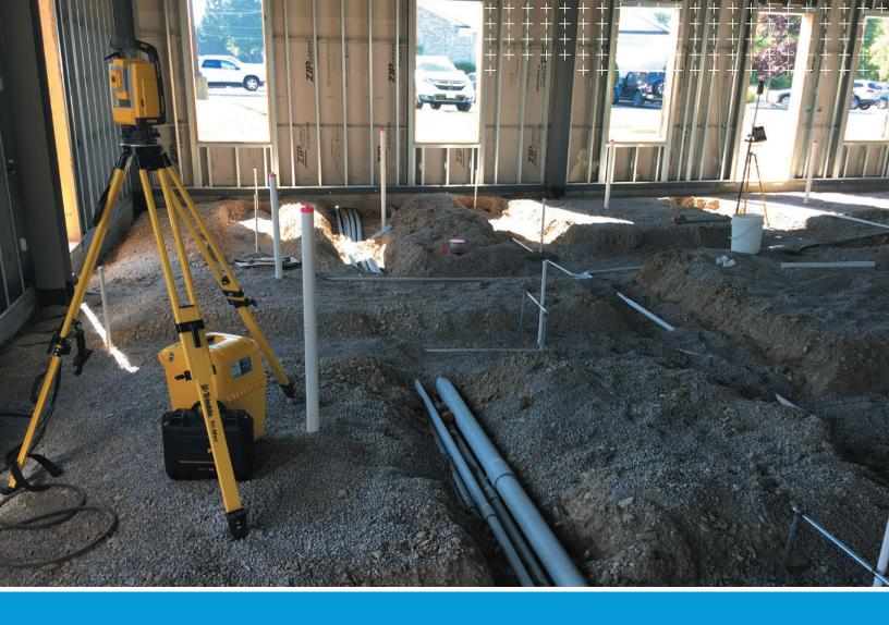
The speed and accuracy of the Trimble X7 3D scanner is helping Warner Mechanical save time and labor resources. What previously took 2-3 days using a tape measure and paper is now easily done in one day.
