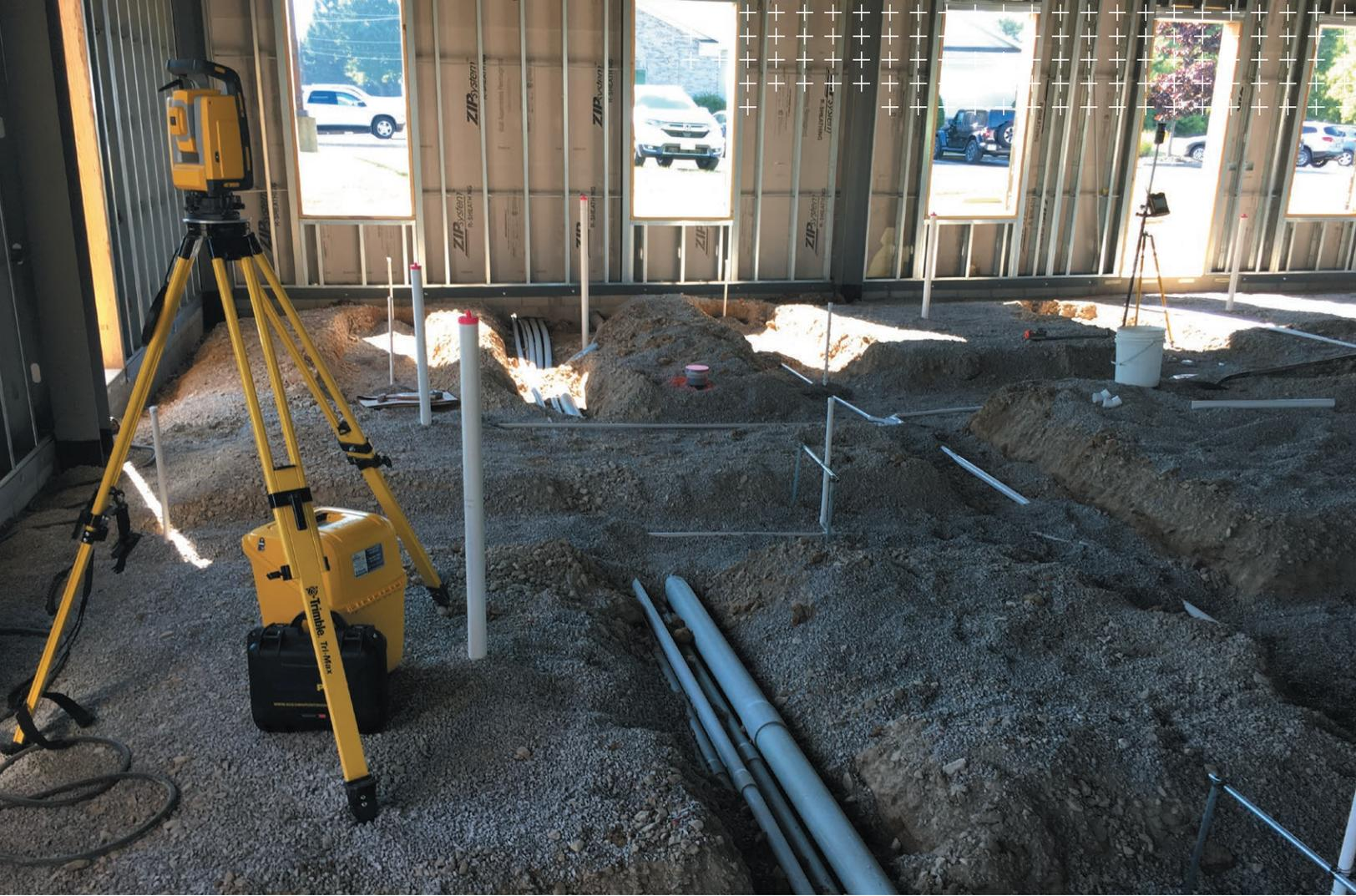
The speed and accuracy of the Trimble X7 3D scanner is helping Warner Mechanical save time and labor resources. What previously took 2-3 days using a tape measure and paper is now easily done in one day.
