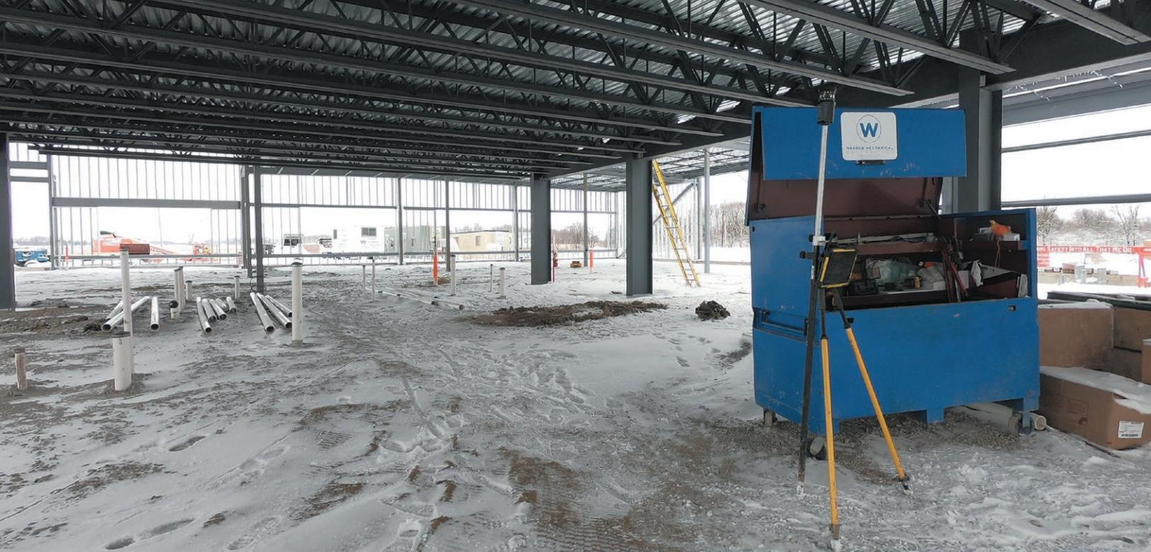
One of Riddell's favorite features of the X7 scanner is the Trimble Registration Assist for in-field registration that allows for automatic scan orientation and alignment with the last pre-selected scan. He also likes the ability to customize the scanner to allow for faster scans and the ability to view both scans and 3D models on the tablet controller for onsite viewing.
